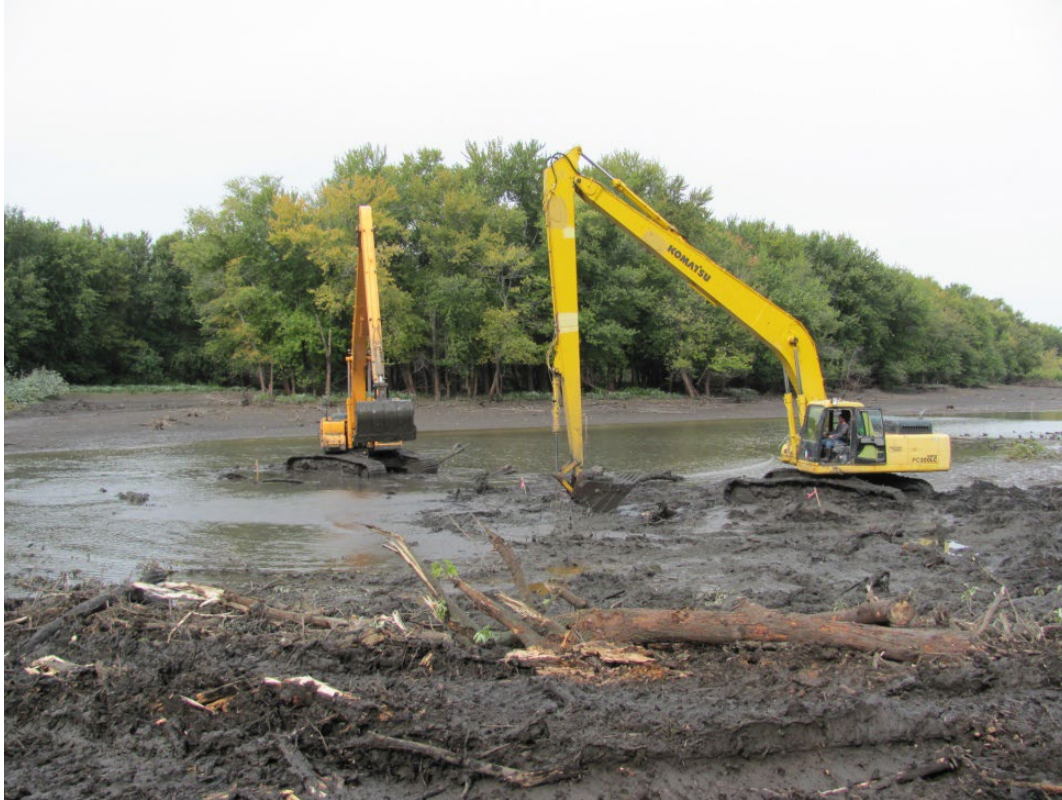
Photograph 3. Marsh Buggy operation Huron Island HREP
